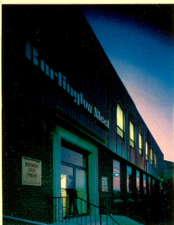
The refurbished Burlington Steel Administration Building.
