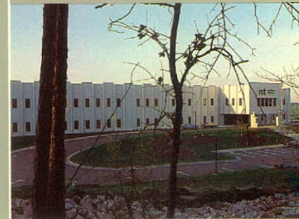
Northern Telecom Inc. officially opened in May 1981 its 250,000-square foot DMS manufacturing plant in Research Triangle Park near Raleigh, N.C. However, the continuing strong demand for DMS switches requires a 76,000-square-foot expansion of the plant which is now underway.
