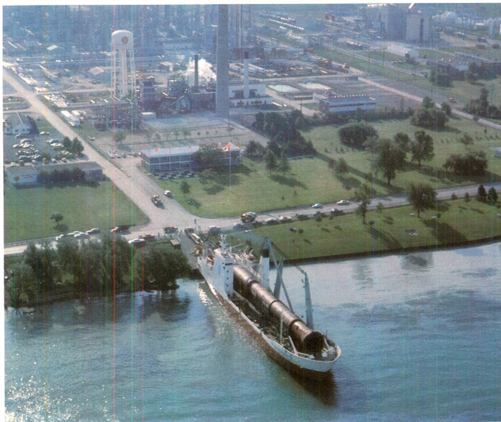
A 20-storey-high splitter tower arrives at Sarnia refinery where it was unloaded at specially designed riverside unloading facilities. The tower will separate propylene product in the polypropylene plant. (Right) A process tower being installed in the expanded aromatics plant at Sarnia.
