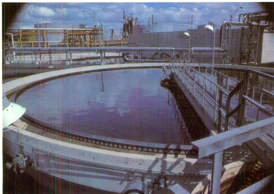
Part of the $22 million effluent treatment plant at Montreal East refinery which went on stream in 1977.
