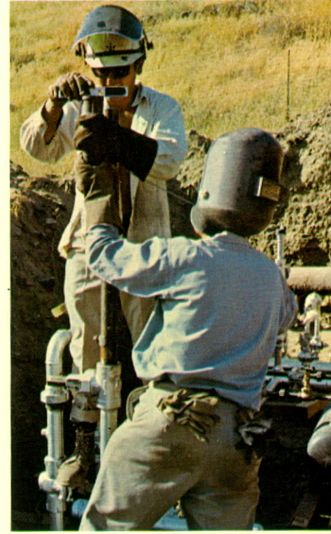
Top left: Welder makes one of three separate welds to complete each joint. Sample joints are x-rayed for quality control.
