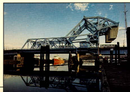
Victoria's sky-blue Johnson Street Bridge, crossing the Gorge Inlet from the downtown core to Esquimalt, was designed by Joseph Strauss, whose other structures include San Francisco's Golden Gate. The 1922 bridge has sections raised by electric motor to permit water traffic to pass beneath.
