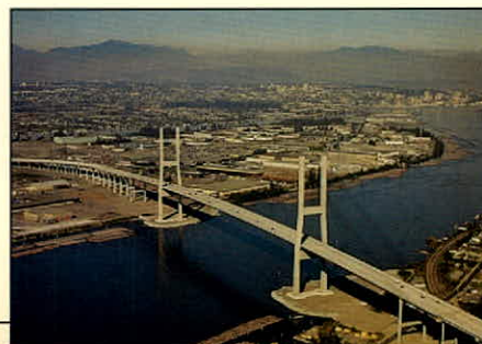
The Alex Fraser Bridge, named for the Minister of Transportation and Highways at the time of its construction, was opened in September, 1986. It is part of a highway/interchange network known as the Annacis System. At 2,500 metres, the Fraser River crossing is the longest cable-stayed structure in the world.
