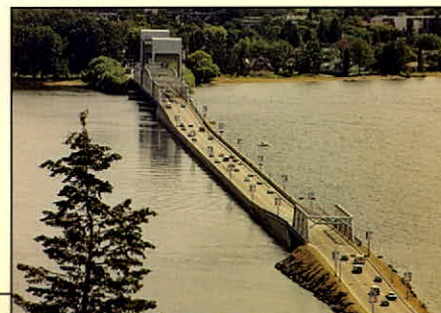
It was the summer of 1958 when Princess Margaret cut the ribbon to open the Okanagan Lake Bridge. That is the formal name of the crossing between Kelowna and the lake's west bank, but it is popularly known as the Okanagan floating bridge. To suit sub-surface conditions, the bridge was designed with floating piers, concrete pontoons and a steel-decked lift span.
