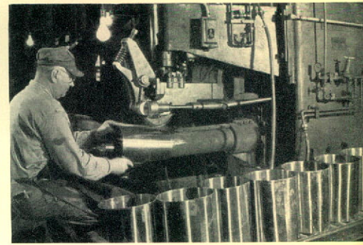
Resistance Welding Milk Can Seams
