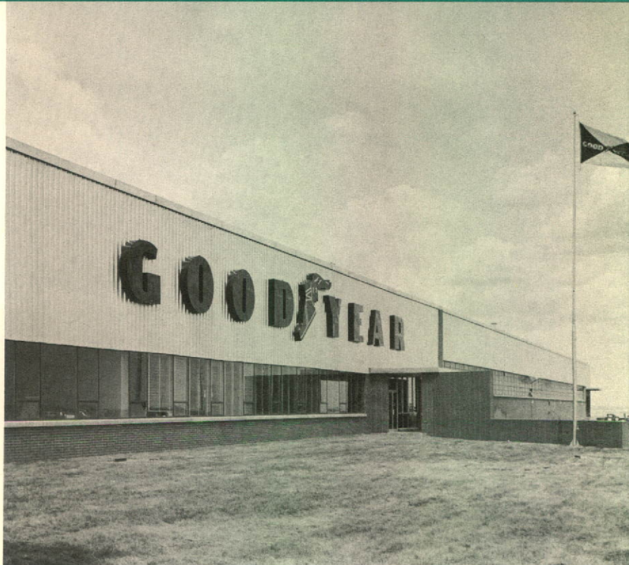
Goodyear Tire & Rubber Company of Canada Ltd. plant, Medicine Hat. Engineers: Fenco.
