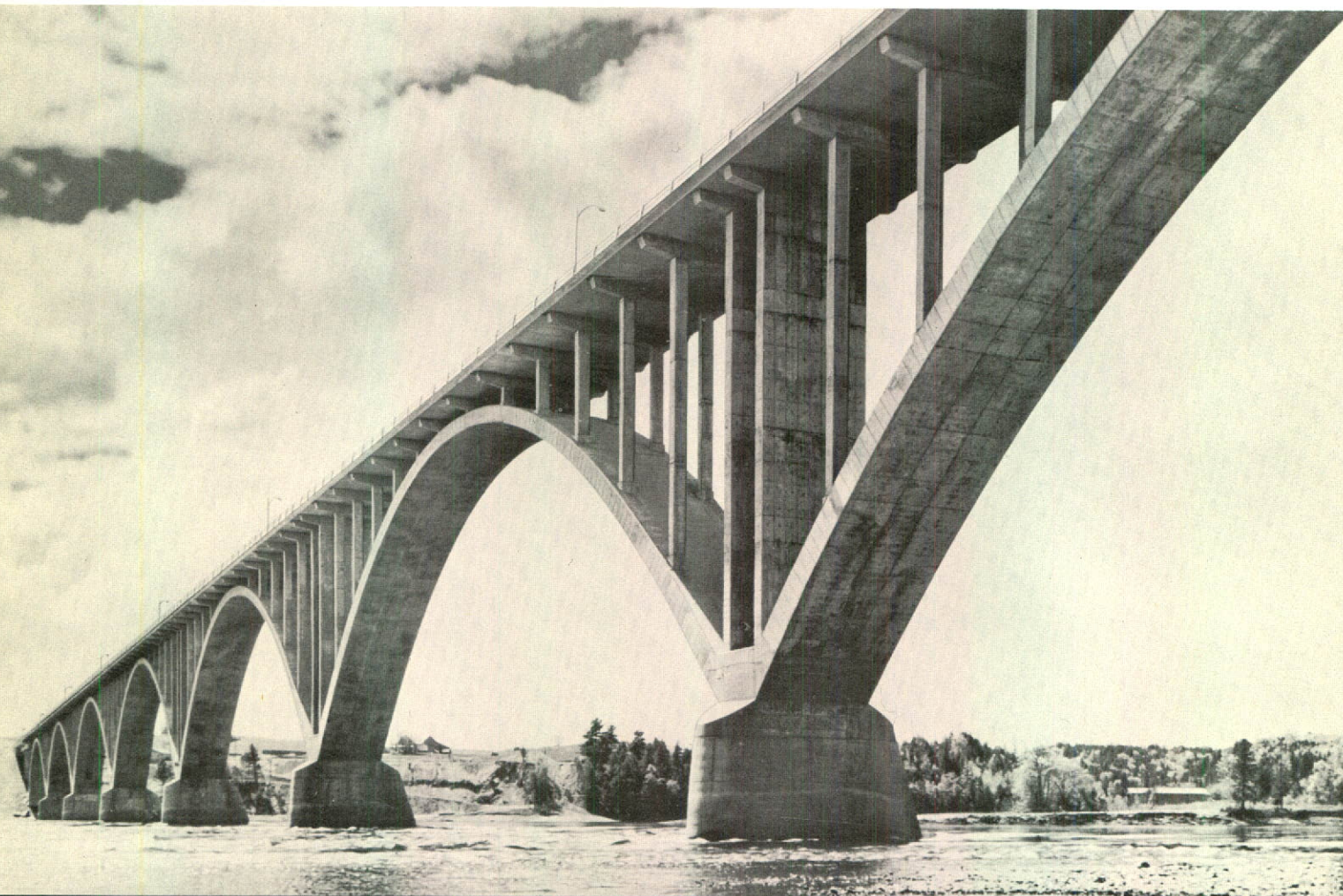
Hugh John Flemming Bridge, Hartland, N.B. Engineers: Fenco for The New Brunswick Department of Public Works.
