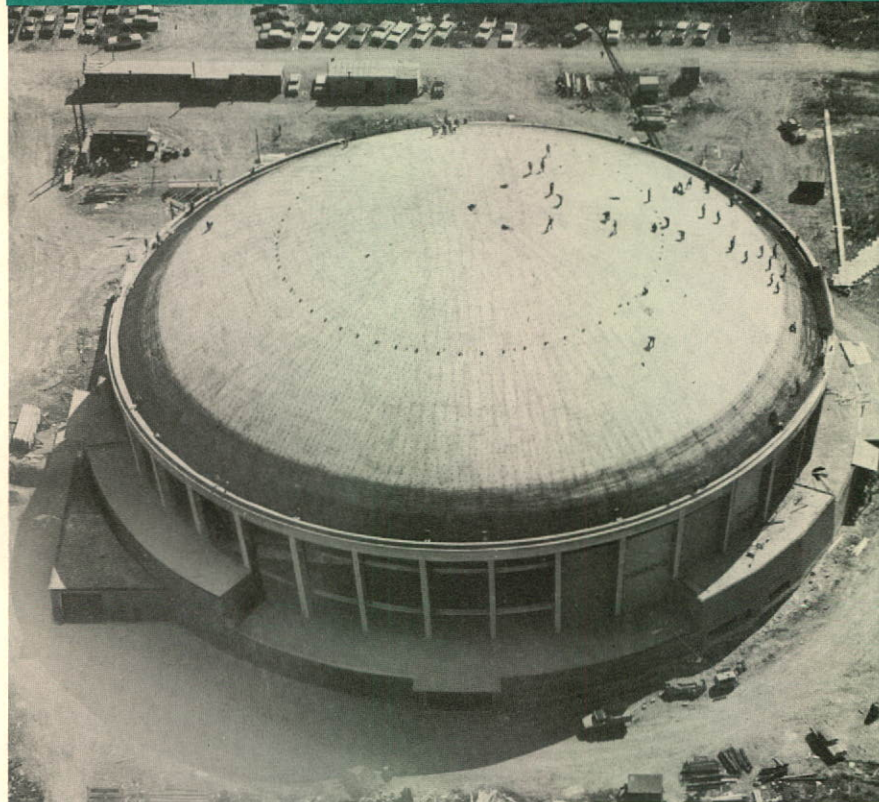
Maurice Richard Arena. Gunite Division subcontracted shell roof from Charles Duranceau Ltée. Architect: Jean Perreault; Structural Engineers: Brouillet & Carmel for Montreal Parks Department.
