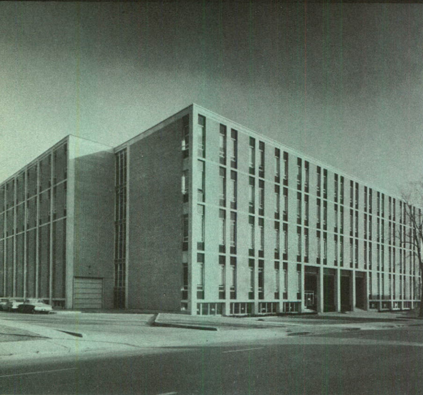
The Galbraith Engineering Building, University of Toronto. Architects: Page & Steele.
