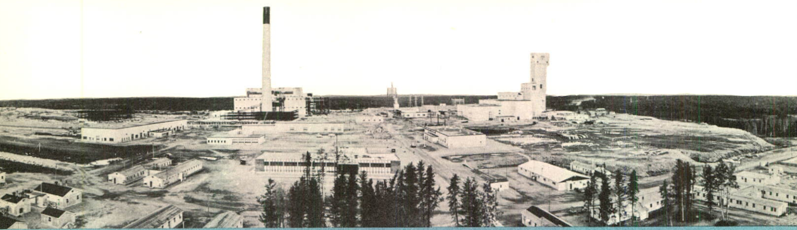
At Thompson, Man., The International Nickel Company of Canada, Limited has taken industrial and resource development deep into the north. Owner's Chief Engineer: N. H. Kearns, B.A.Sc.
