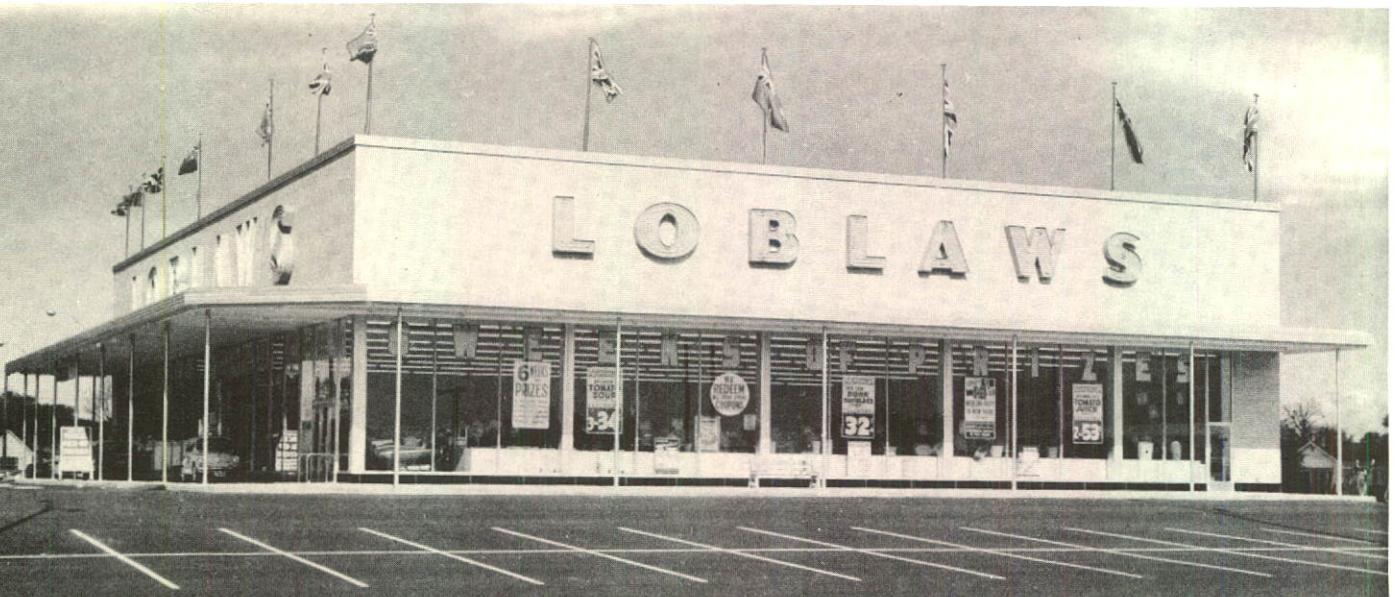
One of many supermarkets built in 1958 for Loblaw Groceterias Co. Limited in various Ontario and Western Canadian towns and cities.
