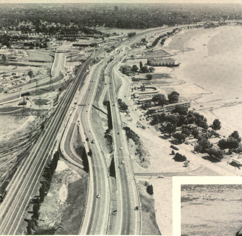
Part of the Frederick G. Gardiner Expressway. Shown are the Humber River bridges, T.T.C. underpass and C.N.R. overpass. Foundation constructed these for the Department of Highways of Ontario, The Municipality of Metropolitan Toronto, Toronto Transit Commission and Canadian National Railways.
