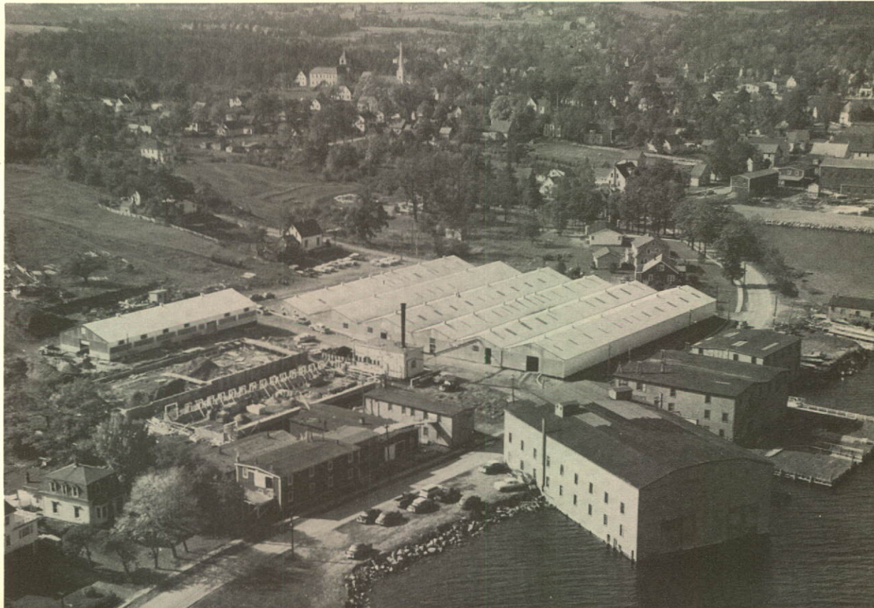
Butler Buildings for Industrial Shipping Ltd., Mahone Bay, N.S.
