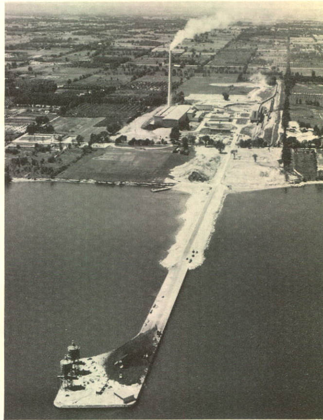
Aerial view of completed 2600 ft. wharf for St. Lawrence Cement Company, Clarkson, Ontario. Designing Engineers: FENCO.
