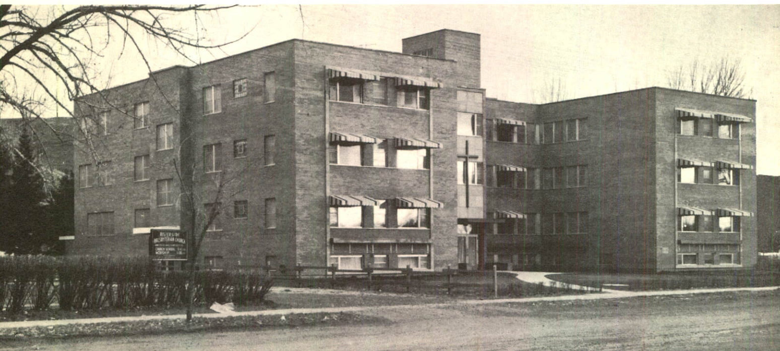
Carmelite Sisters Home for the Aged, Medicine Hat, Alberta. Architects: Rule, Wynn & Rule.
