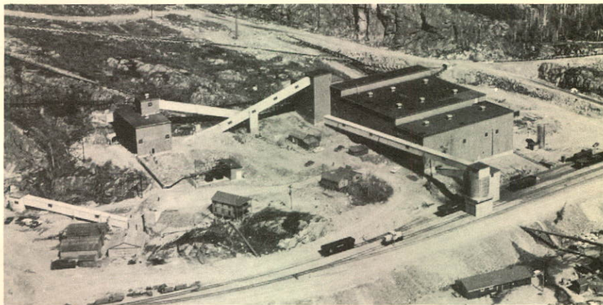
Mill for Falconbridge Nickel Mines Limited, Levack, Ontario. Designing Engineers: FENCO. The large picture shows the installation of Ball Mills.
