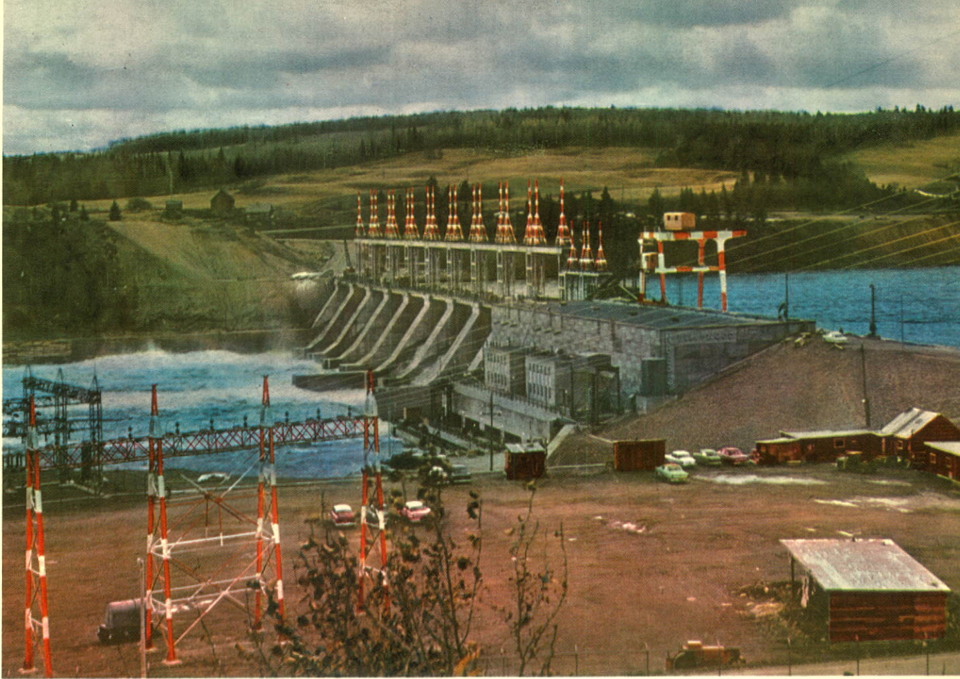
Beechwood Hydro-Electric Development on the St. John River for The New Brunswick Electric Power Commission. Consulting Engineers: Shawinigan Engineering Co., Limited.
