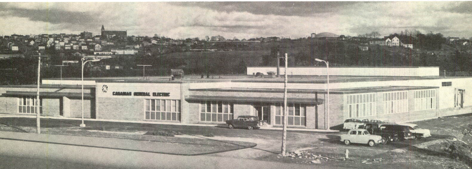
Plant for Canadian General Electric Company Limited, Halifax. Consulting Engineers: Hanks & Irwin.
