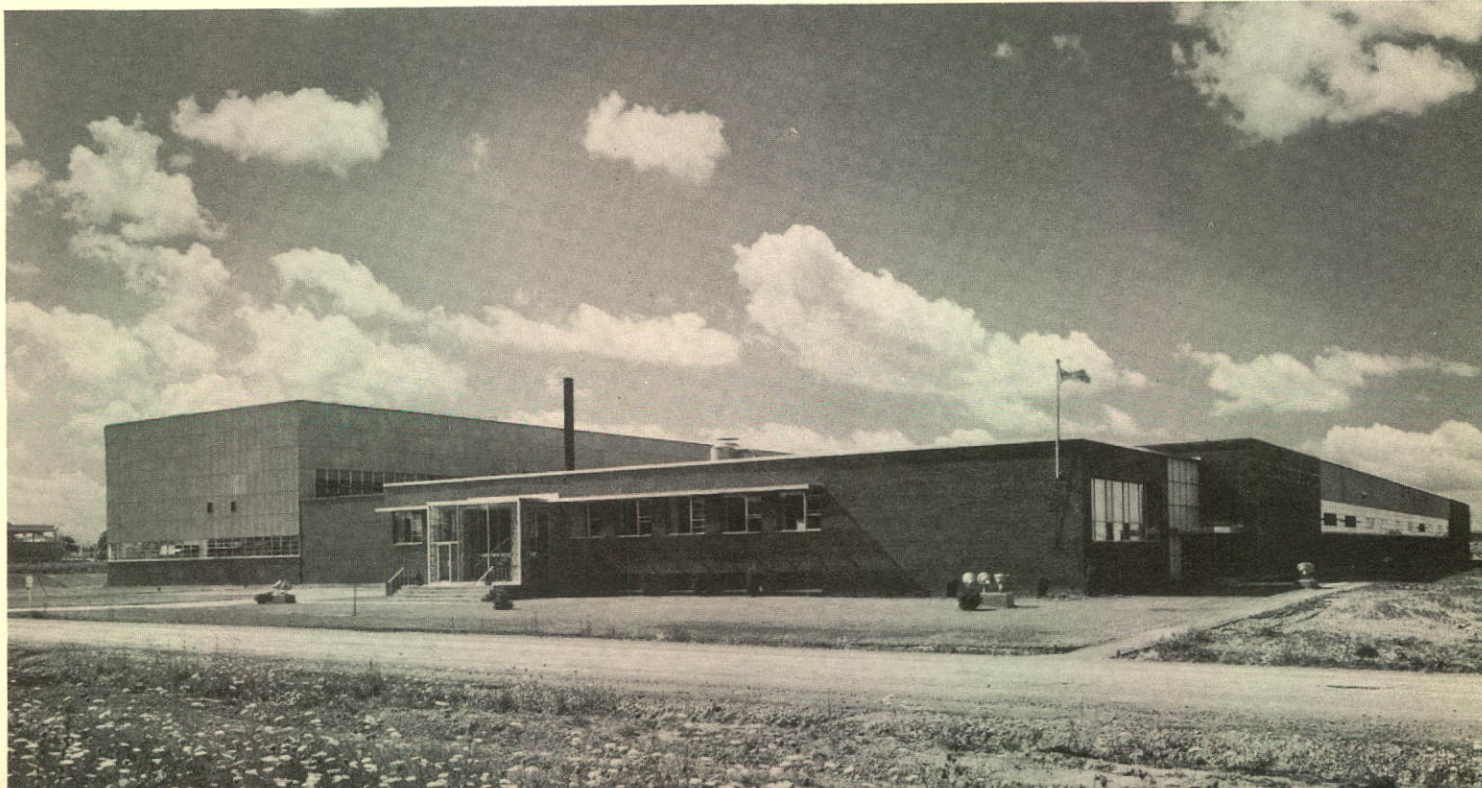
Container plant for Hygrade Containers Limited, Etobicoke, Ontario. Designing Engineers: FENCO.
