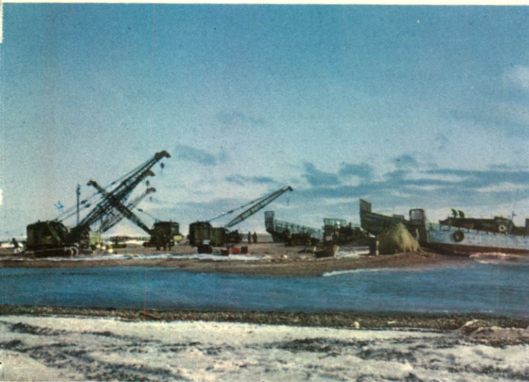
Construction plant being unloaded from landing craft.
