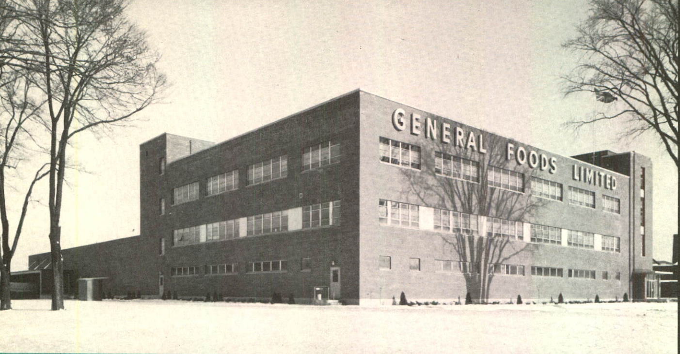
Plant for General Foods Limited, Cobourg, Ontario. Owners' Chief Project Engineer: A. W. Huges.
