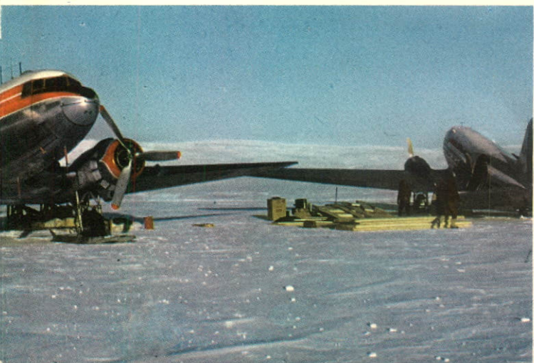
Below: Construction materials arrive at sites in ski-equipped DC-3 Transports.
