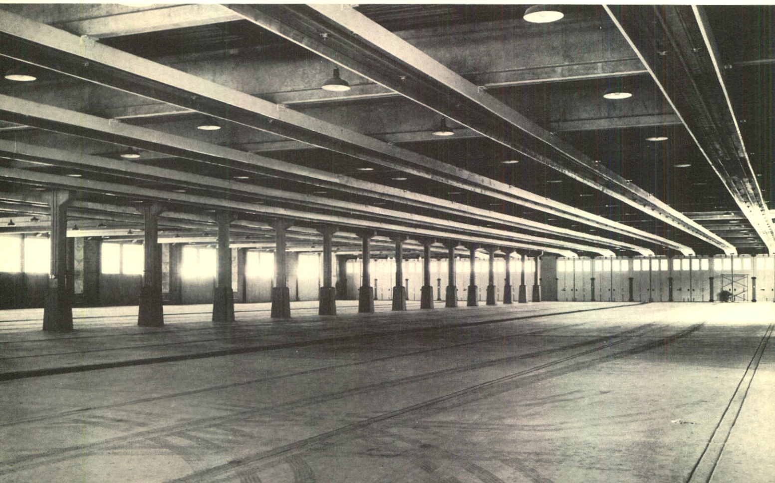
Transit system storage garage for City of Calgary. Consulting Engineers: Haddin, Davis & Brown Ltd.
