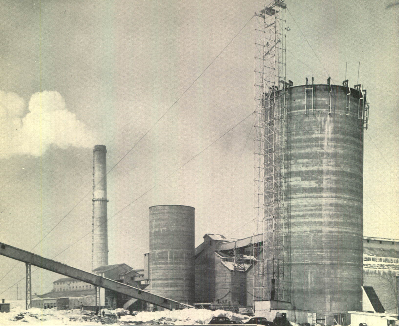
Two 50 ft. x 114 ft. reinforced concrete silos built for Canada Cement Company Limited, Montreal. Owners' Chief Engineer: H. B. Howe.
