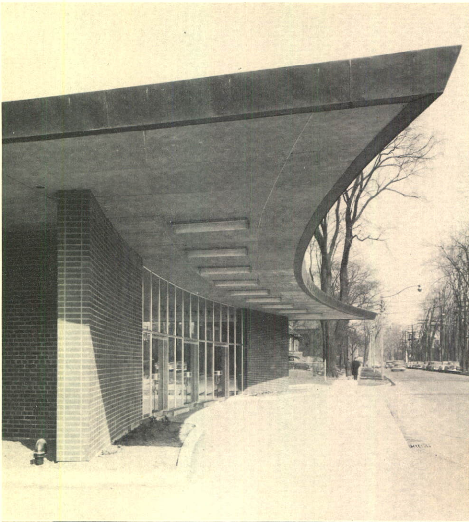
One of the stations of the Toronto Transportation Commission's Subway. Foundation built eleven out of twelve stations.
