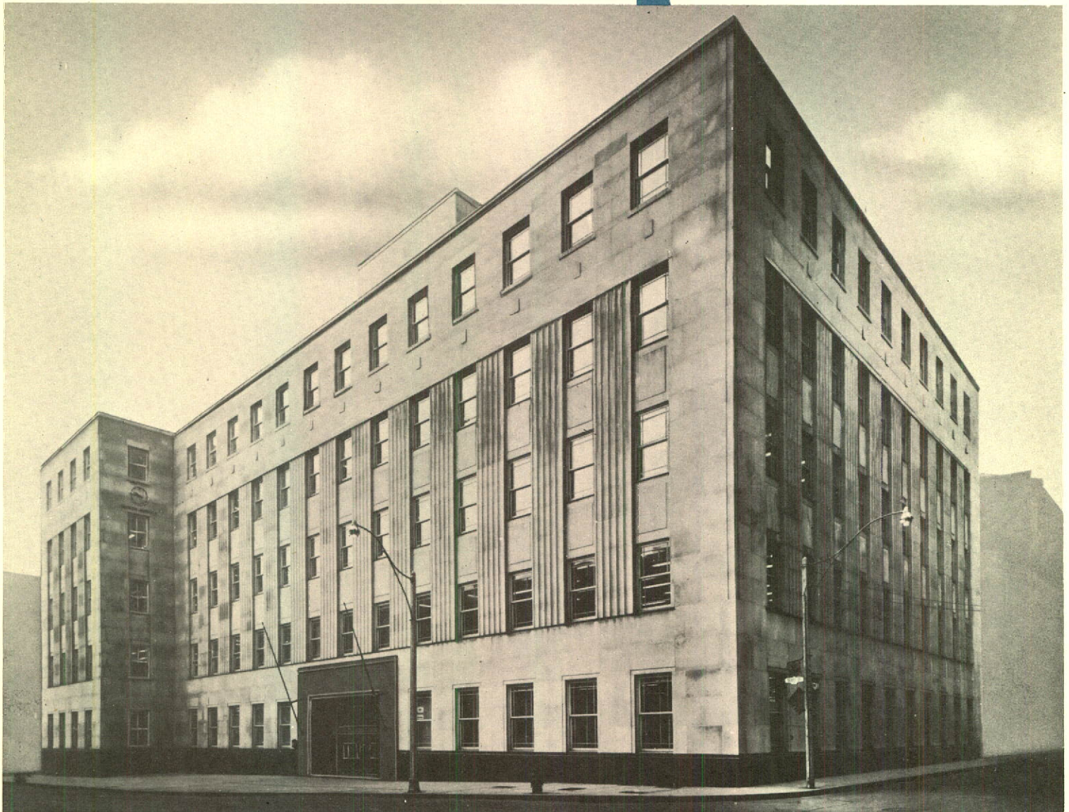
Five-storey Head Office Building. The Western Assurance Company — The British-America Assurance Company, Toronto. Architects: Parrott, Tambling & Witmer.
