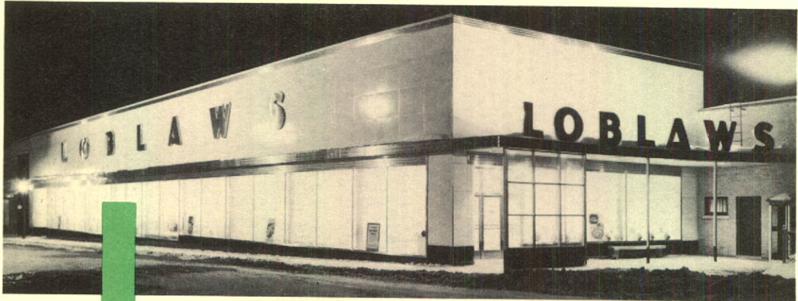
Loblaw Groceteria, Sudbury, Ont. Architects, Parrott, Tambling & Witmer
