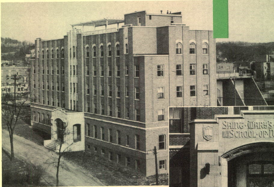
Nurses' Residence, St. Mary's Hospital, Montreal. Architect, E. J. Turcot
