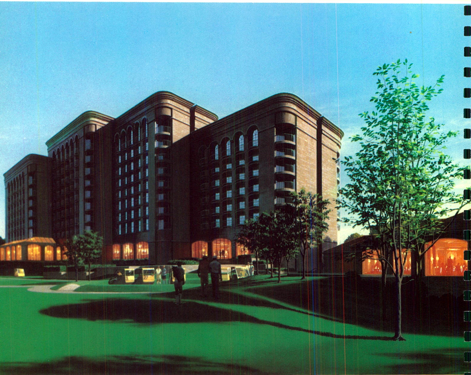
Las Colinas Inn and Conference Center, Dallas, Texas
