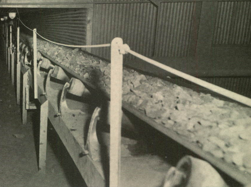
Forano Inclined Belt Conveyor carrying iron ore to the secondary crushers.
