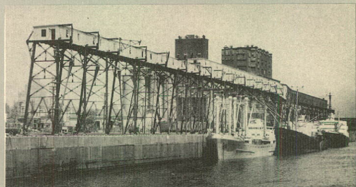
Montreal Elevator features Forano Grain Handling Equipment.
