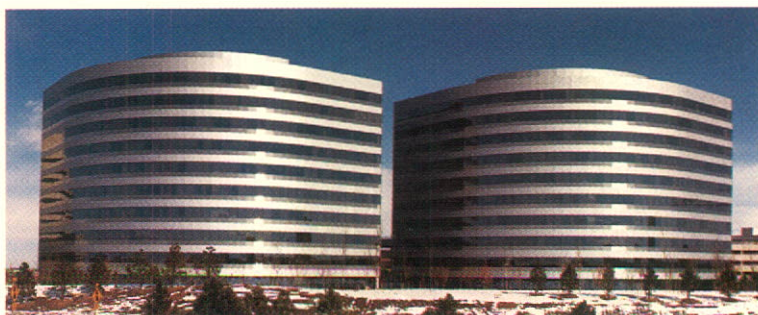
In 1986, Great-West Life completed the second tower of Great-West Life Center, a 460,000 square foot office complex in Denver, housing the Company's United States Headquarters, among other tenants.
