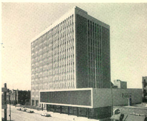
Milner Building — Edmonton.
