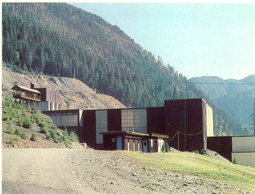
Surface facilities at the Campbell River minesite.
