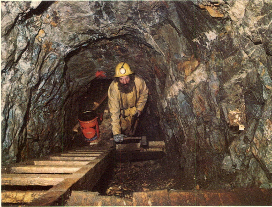
Underground rehabilitation on portion of the promising Big Missouri property where Westmin has encountered encouraging gold/silver potential.
