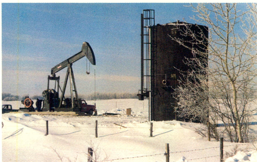
Pump jack and storage tank on Lindbergh heavy oil site.
