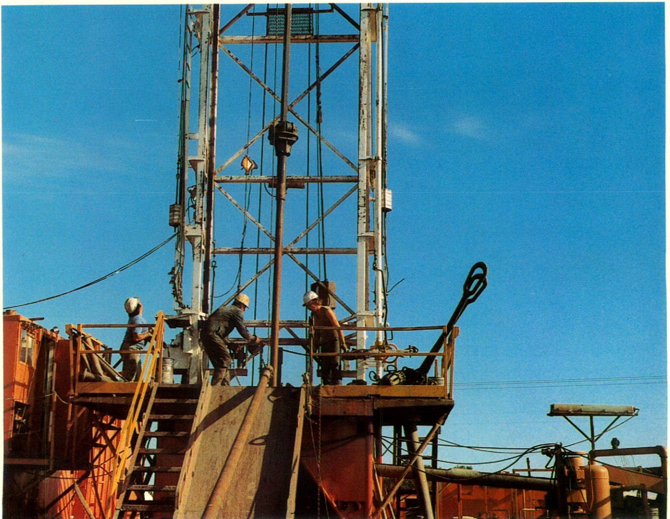
Drilling rig in action.
