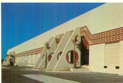
Kyrene Distribution Centre, Phoenix
