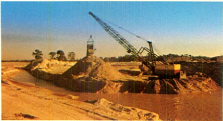
Lake excavation, Boca Pointe
