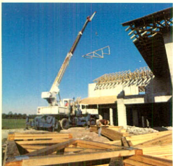
Construction of the golf clubhouse, Boca Pointe
