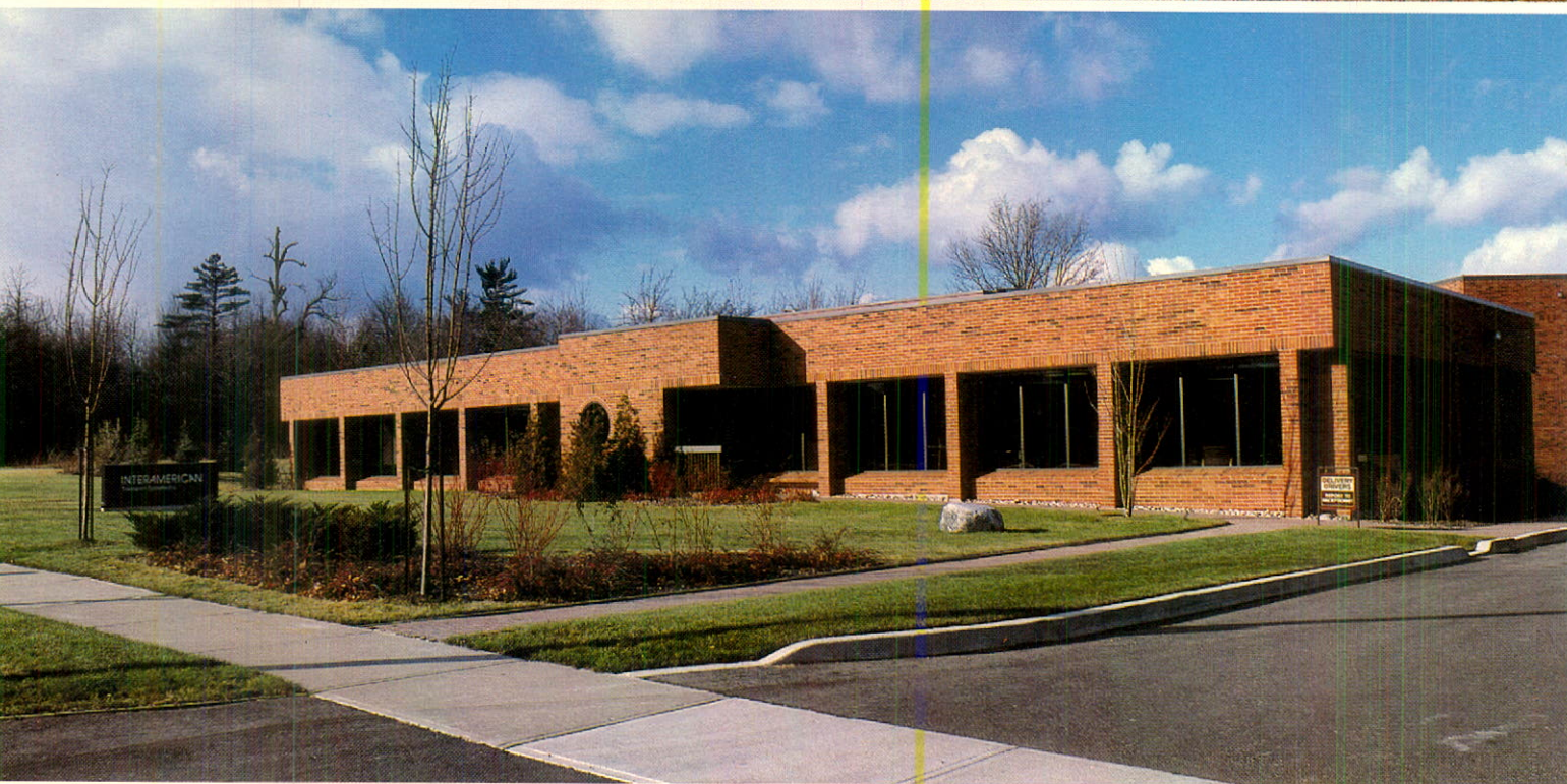
Above: Abbott Laboratories and Interamerican Transportation Systems, developments in the Meadowvale Business Park, Metropolitan Toronto
