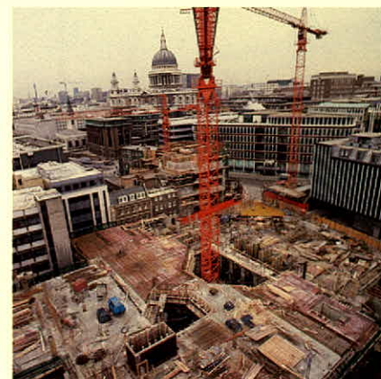
CONSTRUCTION ON THE BEAVER HOUSE SITE, LONDON, ENGLAND
