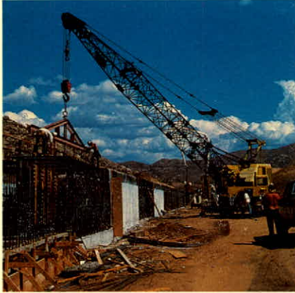
CONSTRUCTION OF THE LAKE SPILLWAY AT SUNNYMEAD RANCH, CALIFORNIA.
