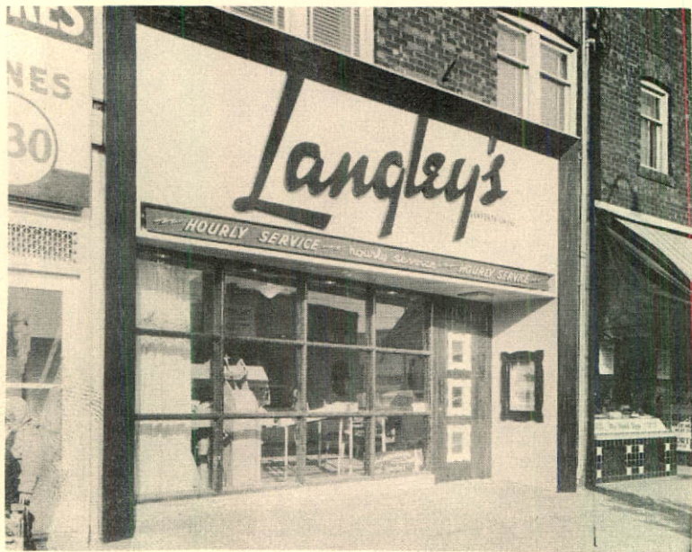
ENTRANCE AT RIGHT is set in 4½ feet, compared with lefthand side. Shirt unit is on constant display just inside front window.
