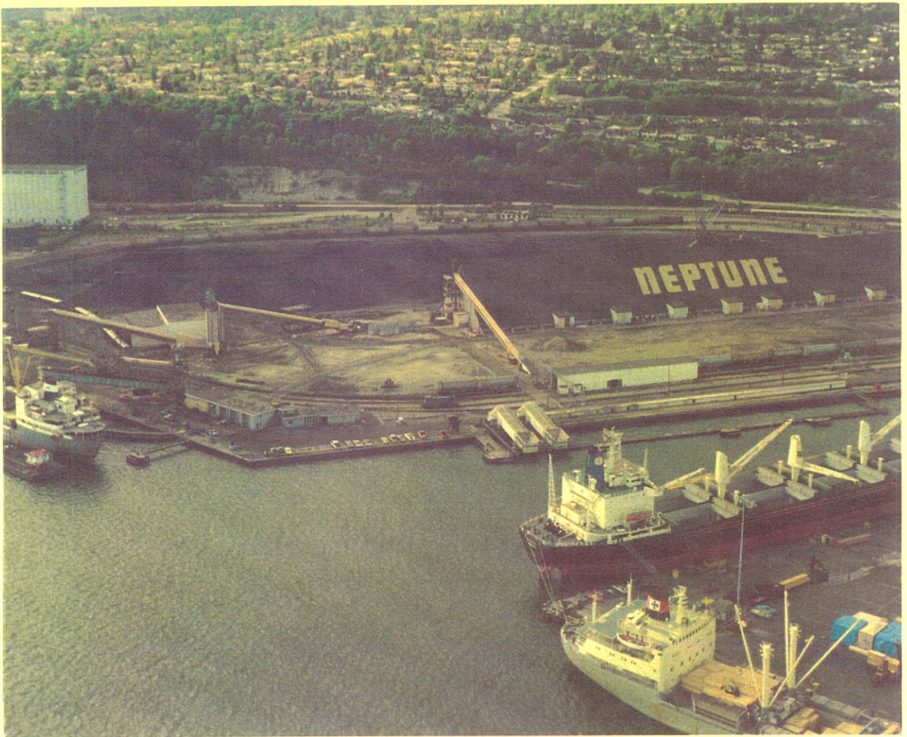
Coal Handling Facilities at Neptune Bulk Terminals (Canada) Ltd.
