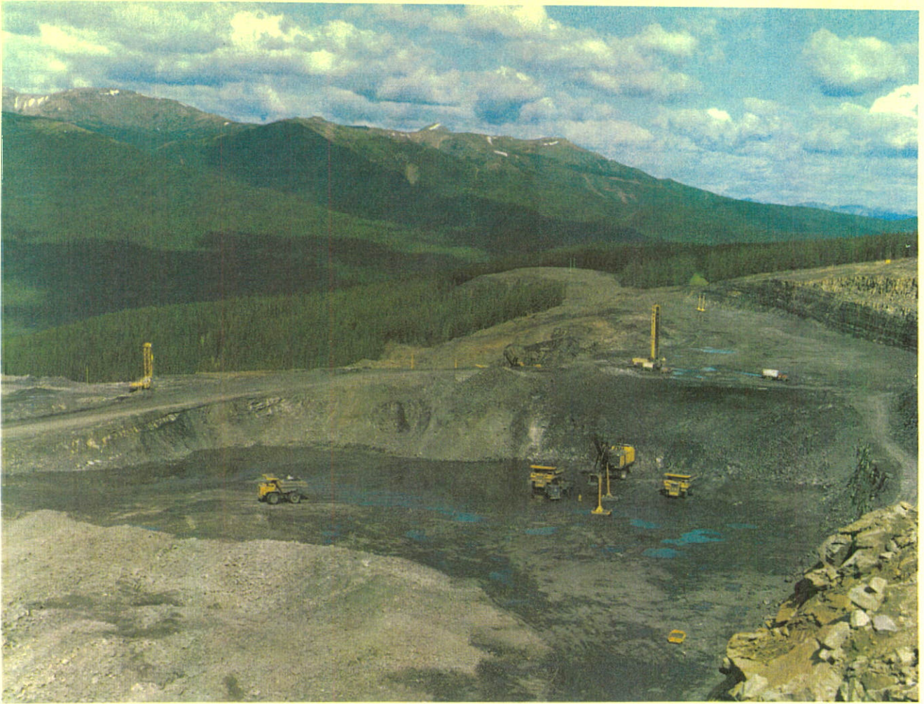
Overburden Removal at #9 Surface Mine
