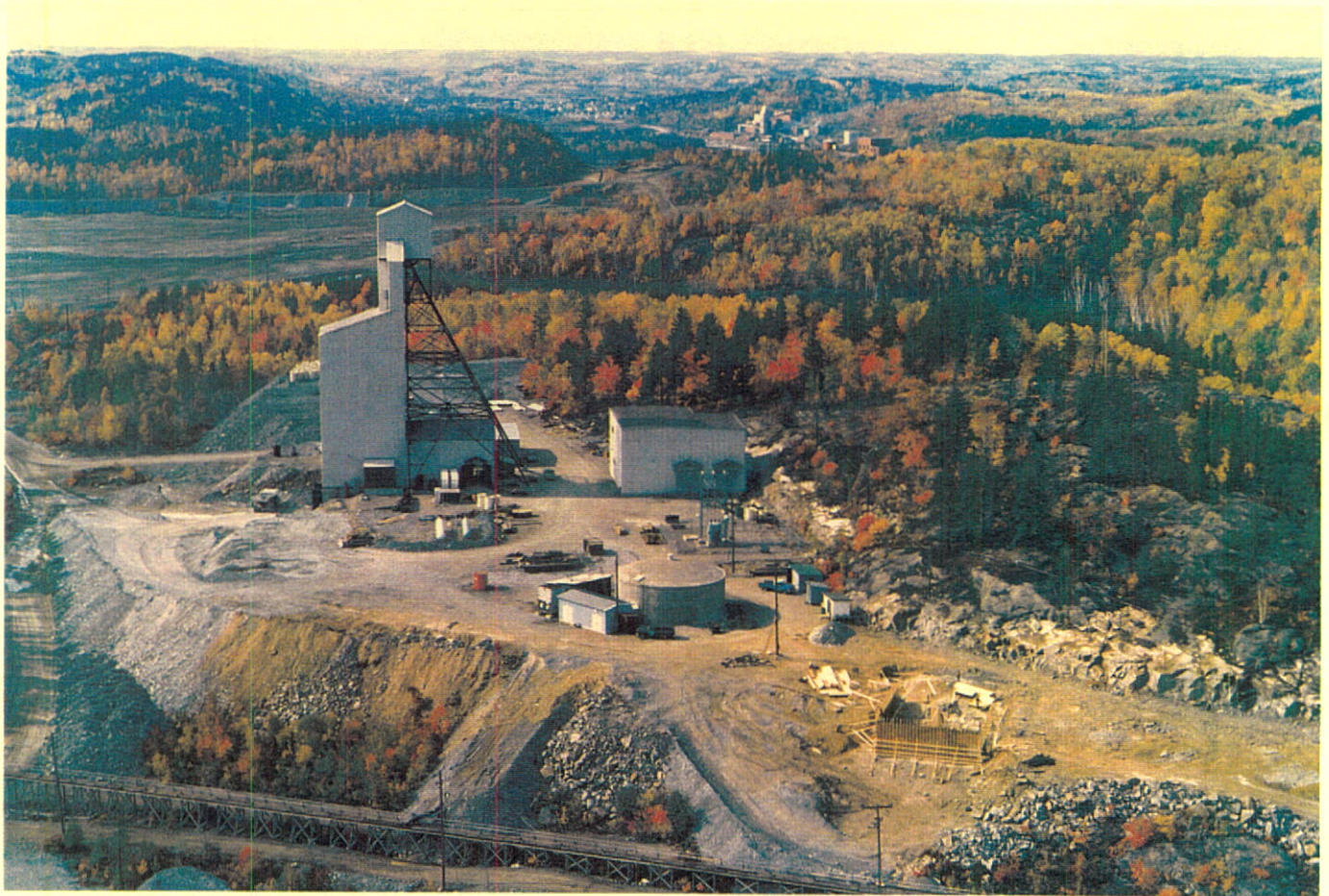
Fraser Mine in the Onaping Area of Falconbridge Nickel Mines' Sudbury operations
