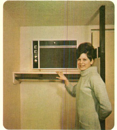
Installation of individual electric room-cooling units assures comfort in hot summer weather.
