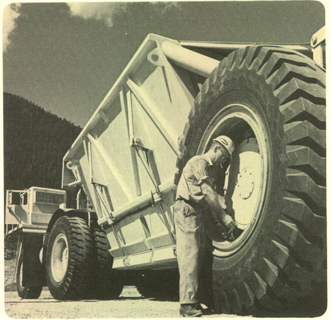
Fill for Mica Dam is hauled by huge 120-ton bottom-dump trucks.
