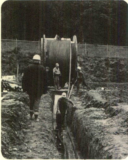
Work started on 11-mile underground extension of 230 kv ring serving Vancouver.
