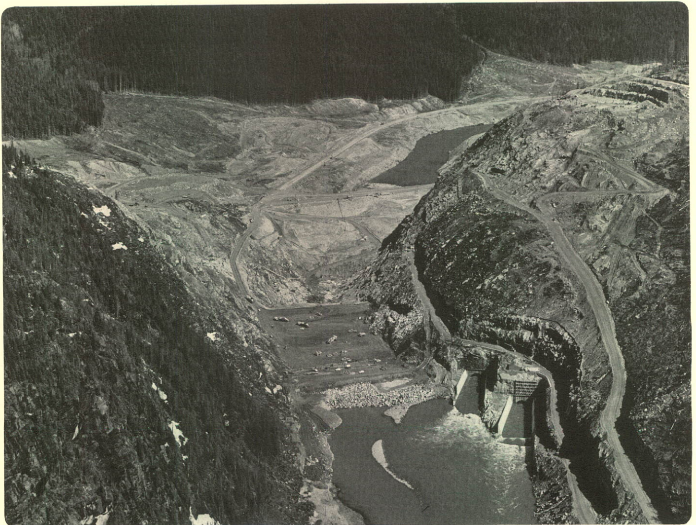
Mica Dam, the final Columbia River Treaty storage project to be completed by the Authority, will rise 645 feet above the riverbed.
