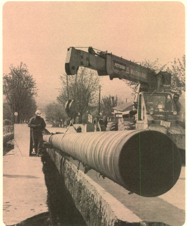
New 20-inch main will make more gas available to the North Shore.
