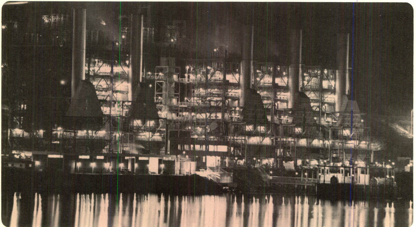
Fourth 150,000 kw generator went into service at Burrard Thermal Generating Plant in September 1967. A fifth unit is now being installed.
