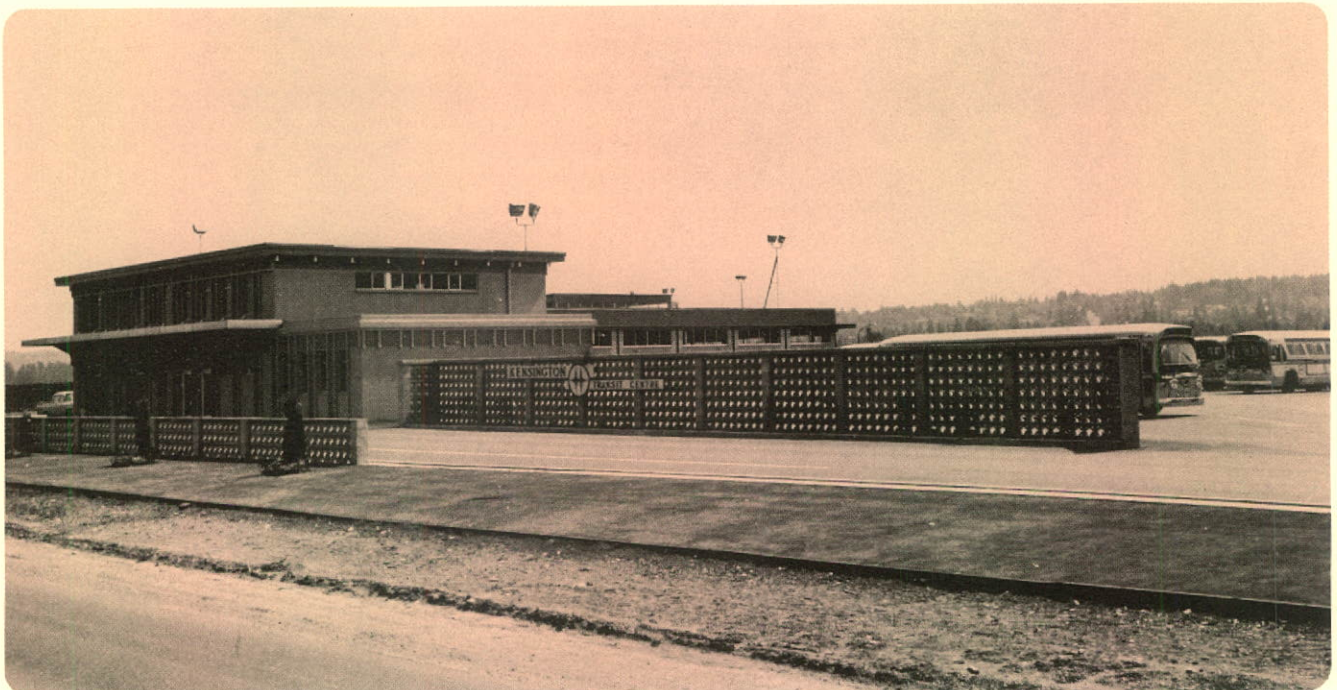
Kensington Transit Centre in Burnaby, opened in June 1967, services urban buses operating in eastern portion of Greater Vancouver.
