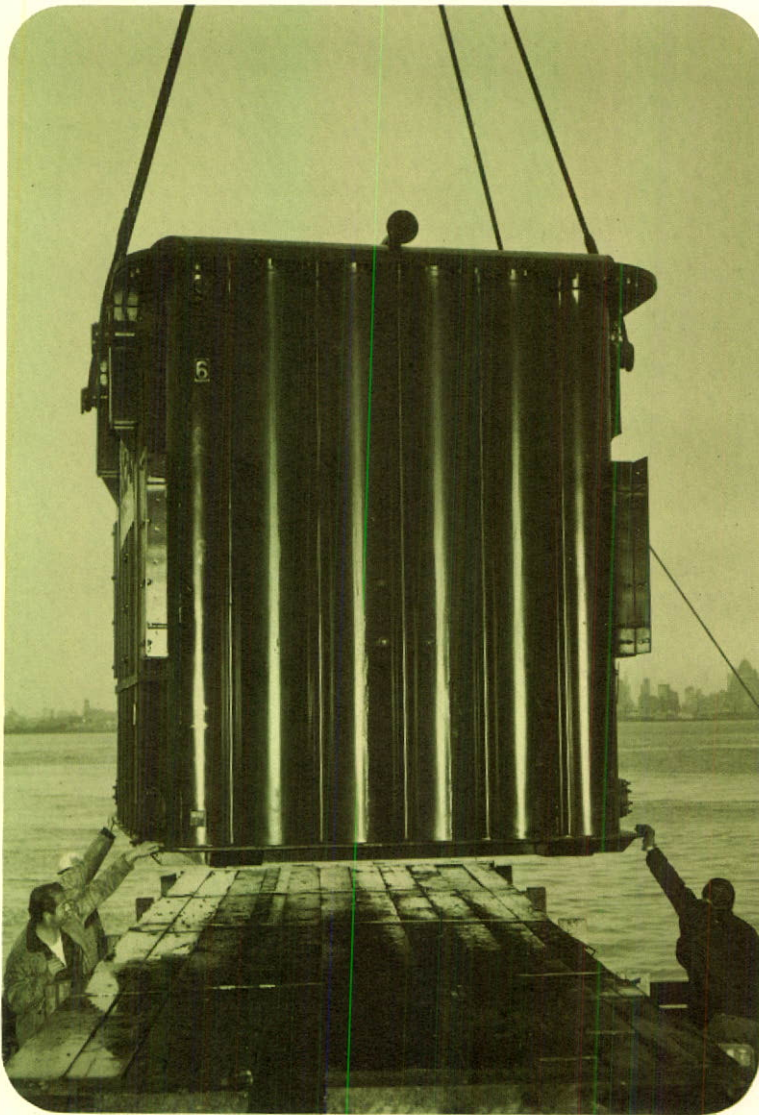
75-ton smoothing reactor en route to Vancouver Island terminal of a high voltage direct current interconnection with the Lower Mainland system.
