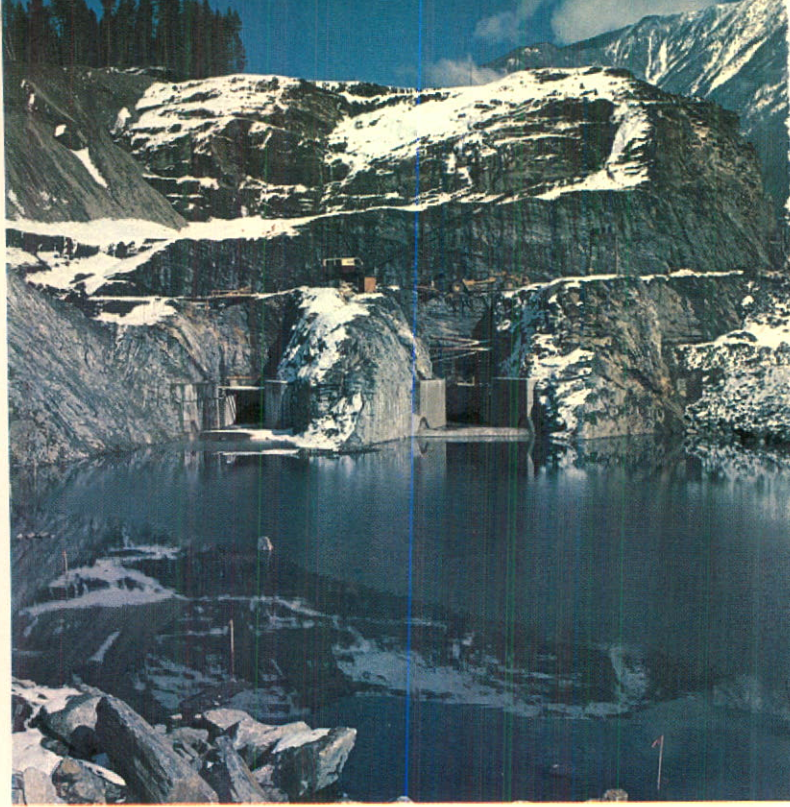
Diversion Tunnels, Duncan Storage Project.
