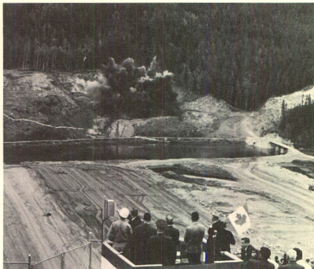
Duncan Project: Rock blast at ceremony marking commencement of major construction.
