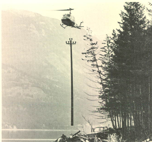
Helicopters facilitate line construction in mountainous terrain of British Columbia.
