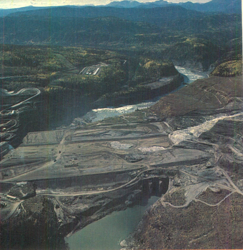
Portage Mountain Dam, Peace River Project.
