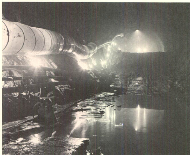
Mica Project: Diversion tunnel No. 2 under construction.
