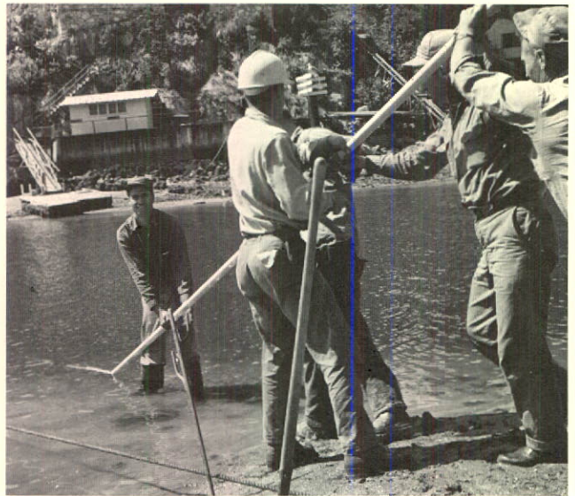
The Authority's first natural gas pipeline under salt water, serving Eagle Island, West Vancouver.
