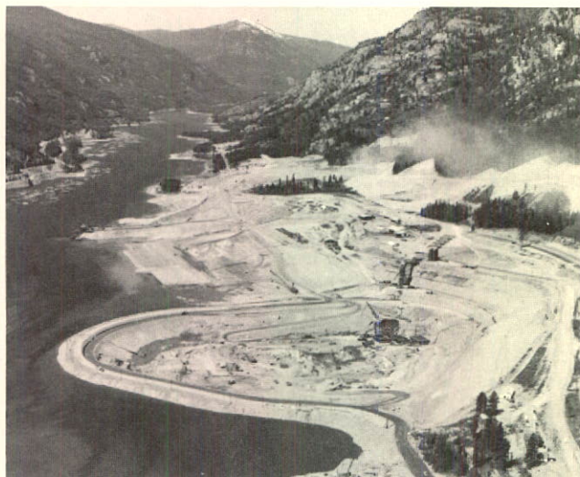
Arrow Project: Upstream view of the Columbia River showing completed cofferdam.
