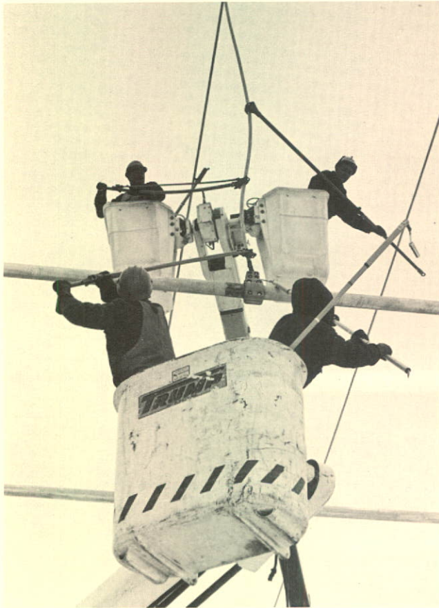
Hot-line crew replacing live 230 kv risers at Williston Substation, Prince George.
