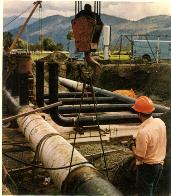
Regulator station at Huntingdon, where B.C. Hydro takes 95% of natural gas purchased from Westcoast Transmission Company Limited, was rebuilt to increase its capacity by 53%.
