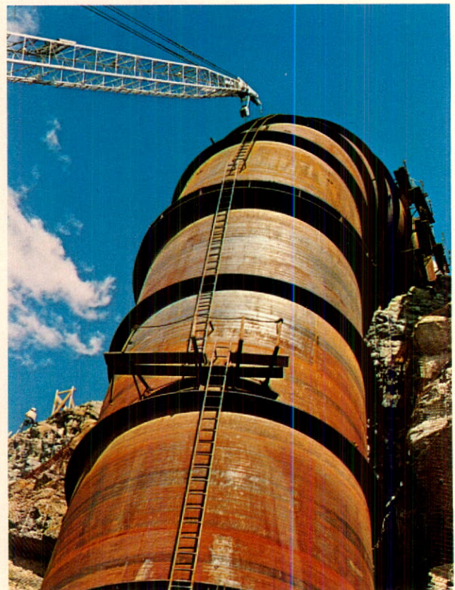
Giant penstocks will feed water to new Kootenay Canal generating plant when it begins operation later in 1975. Two 125,000 kw units at this hydroelectric project will be placed in service in 1975, remaining two in 1976.
