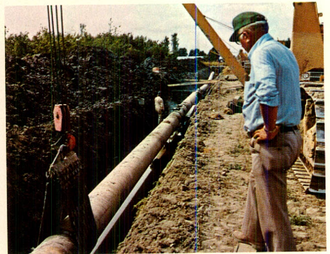
Gas transmission pipeline loop was completed in Richmond.
