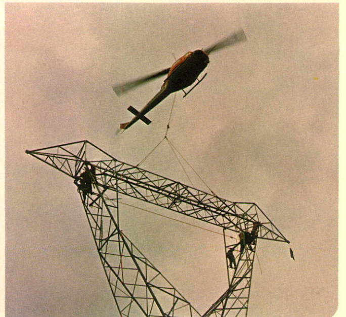
Helicopter lowers sections of transmission tower to waiting workers, who fasten steel components securely into place. Aerial approach was adopted to avoid disturbing terrain where powerline crosses golf course in Surrey. The line is one of the 500,000-volt connections which will deliver power from the Mica project to centres where electricity is needed.
