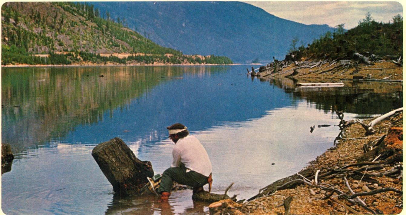
Topping stumps to reduce boating hazard is part of Hydro's foreshore beautification program in Upper Campbell reservoir.
