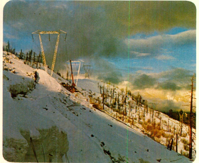
Giant snowslide east of Lillooet knocked out five towers on transmission line from Peace River in January. Crews braved severe weather and rough terrain to repair damage.
