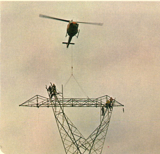
Helicopter lowers sections of transmission tower to waiting workers, who fasten steel components securely into place. Aerial approach was adopted to avoid disturbing terrain where powerline crosses golf course in Surrey. The line is one of the 500,000-volt connections which will deliver power from the Mica project to centres where electricity is needed.
