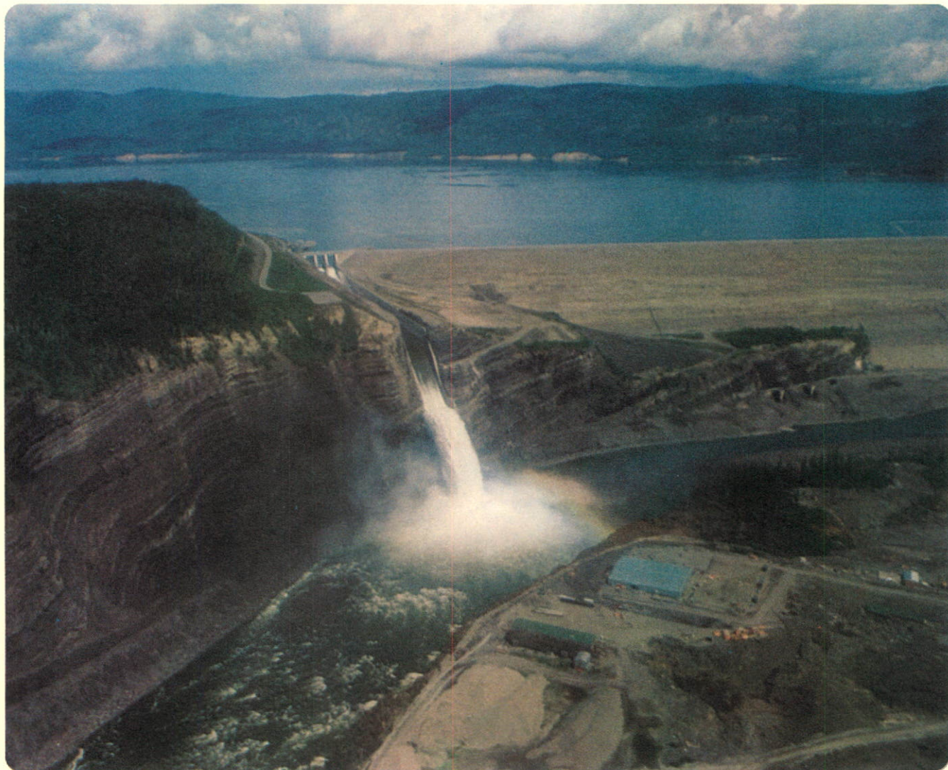
Surplus water, stored in Williston Lake to regulate flow during 1972 flood season, later is released through spillway.
