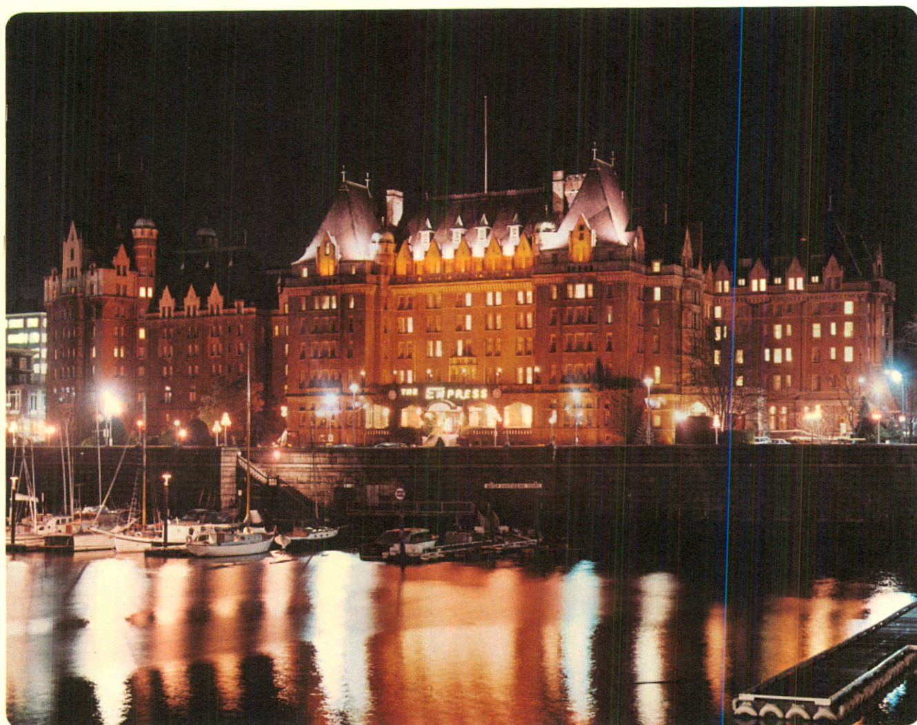
Award-winning outdoor lighting display, designed by B.C. Hydro staff for Empress Hotel, brightens Victoria's Inner Harbour.
