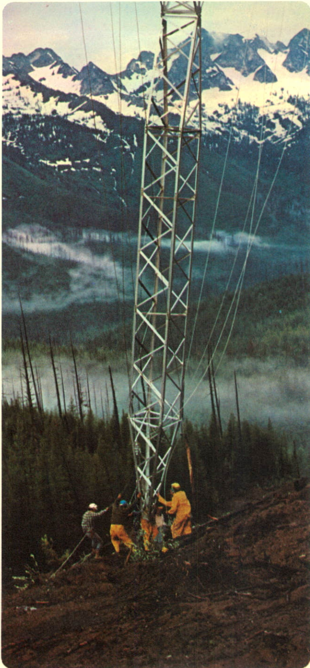
... to right-of-way where workmen secure them into place.
