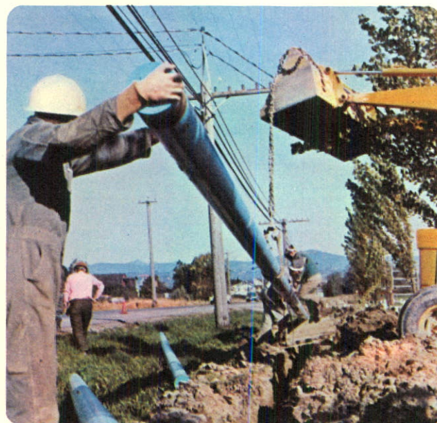
Section of new line is placed in trench north of Matsqui.
