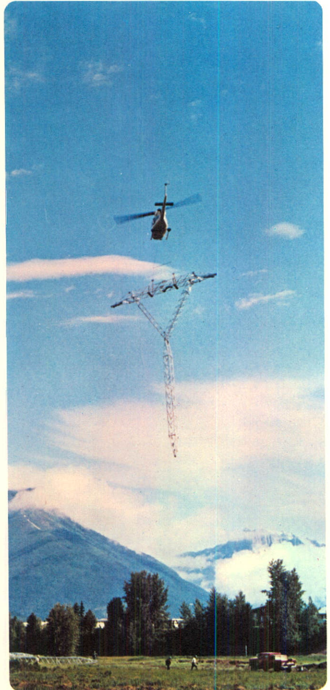
Helicopter takes towers for Cranbrook-Natal power line . . .
