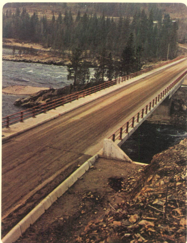
Access bridge leads to construction site at Kootenay Canal.
