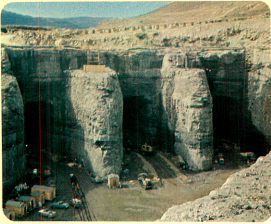
1962 — Diversion tunnels for Peace River Project.
