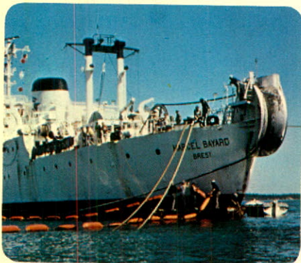
1969 — Cable-laying for HVDC intertie.
