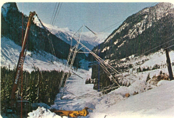
Emergency line repairs near Squamish ended power crisis.
