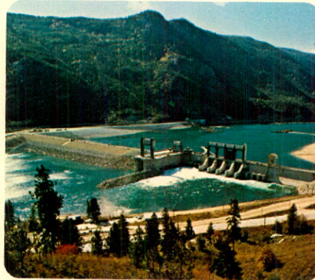
1968 — Hugh Keenleyside Dam in service.
