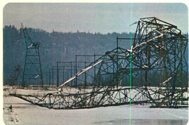
Temporary line was built to replace damaged section.
