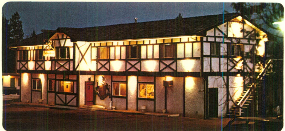
Effective use of outdoor lighting is demonstrated at motor hotel in Williams Lake.
