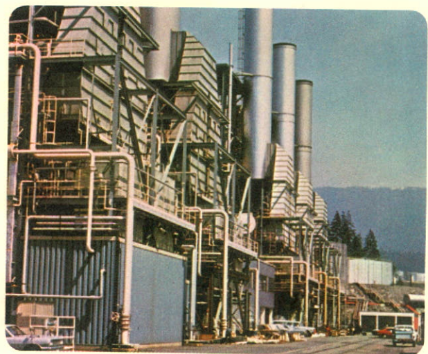
Acoustical barriers to dampen noise from boiler fans are being installed at Burrard Thermal Generating Plant.
