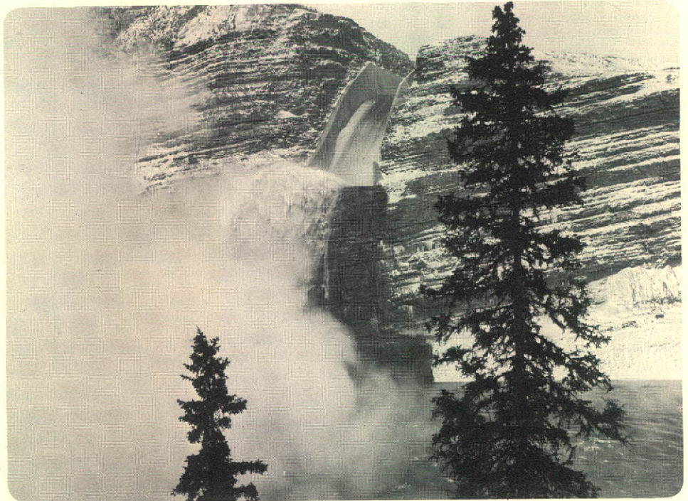
Water cascaded down W.A.C. Bennett Dam spillway for first time during test in 1970.
