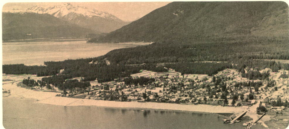
Unique soil cement protection for waterfront, built by B.C. Hydro at Nakusp, is an important side benefit to the community from construction of Arrow storage project.
