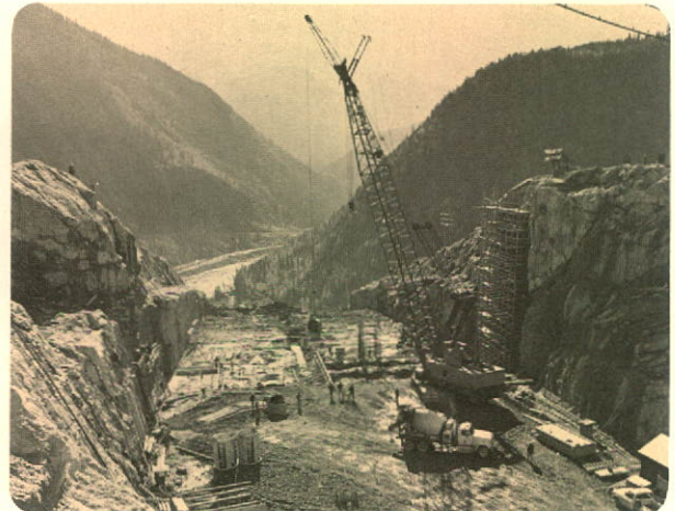
Excavation for Mica Dam spillway progressed steadily.
