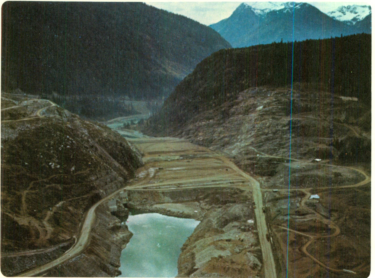
Mica Dam, last Columbia Treaty storage project to be built by B.C. Hydro, will be highest earthfill dam on continent.
