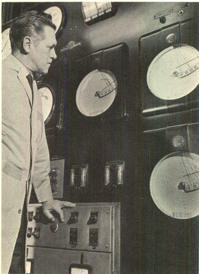
Smoke density recorders indicate efficiency of combustion.
