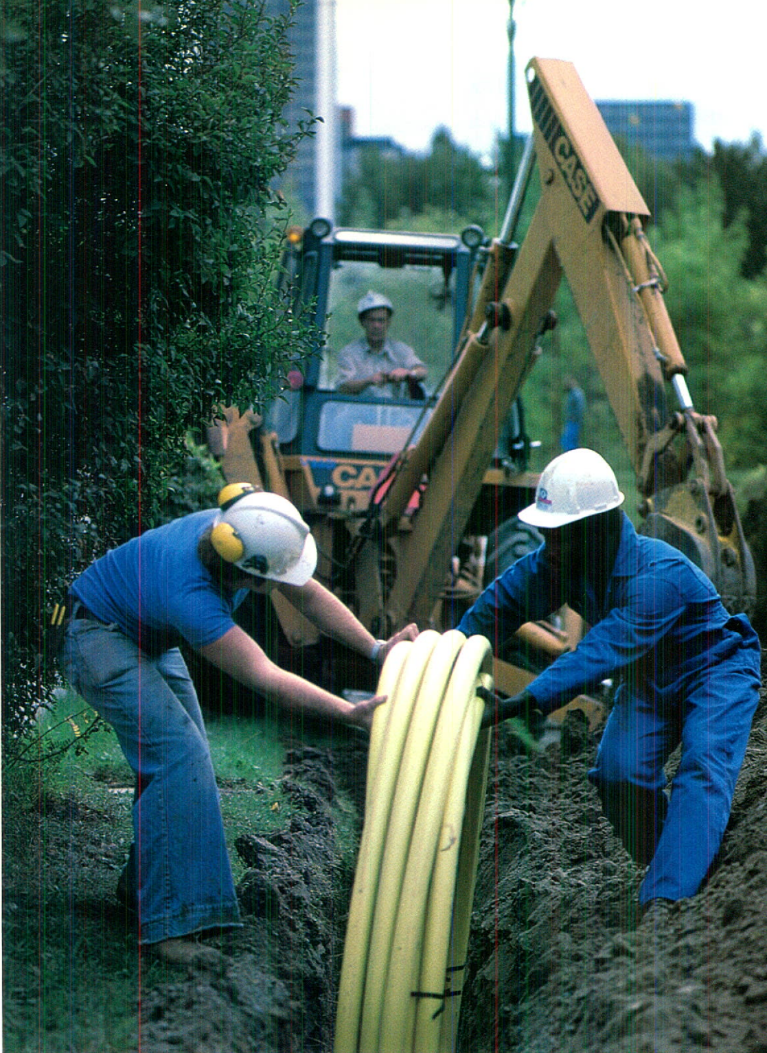
Canadian Western and Northwestern answered 128,975 customer service requests during 1981 (above left). Plastic pipe was introduced for urban natural gas distribution (above right) while this NUL valve assembly at Viking Camp improves deliverability of gas from the Viking Field (below right).
