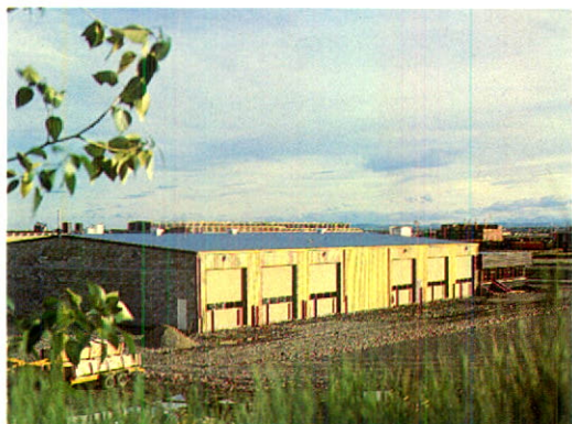
A truck maintenance shop owned by Crone Bros. Ltd., Calgary, built of structural steel and cladding manufactured by ATCO Metal.
