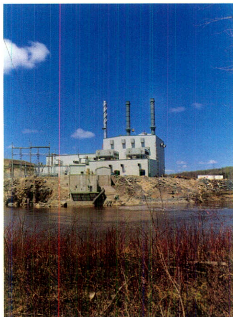
ATCO Noise Management designed, supplied and constructed the acoustic envelope for Northland Power's 104 MW cogeneration plant at Iroquois Falls, Ontario.
