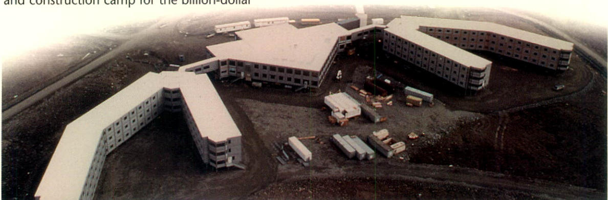
The three-storey, 165,000 square foot permanent accommodation facility for the Falconbridge Raglan Project in northern Quebec accommodates 300 people.
