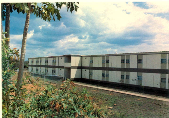
700-man ATCO housing complex supplied to Venezuelan government electrification agency.
