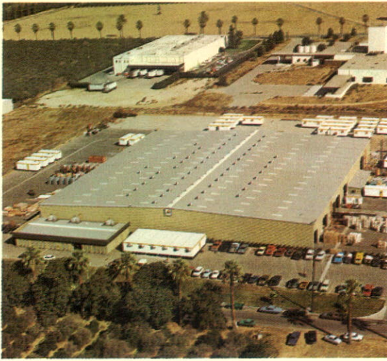
Left: One of ATCO International's modern manufacturing facilities.
