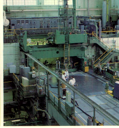
NRU Research Reactor
