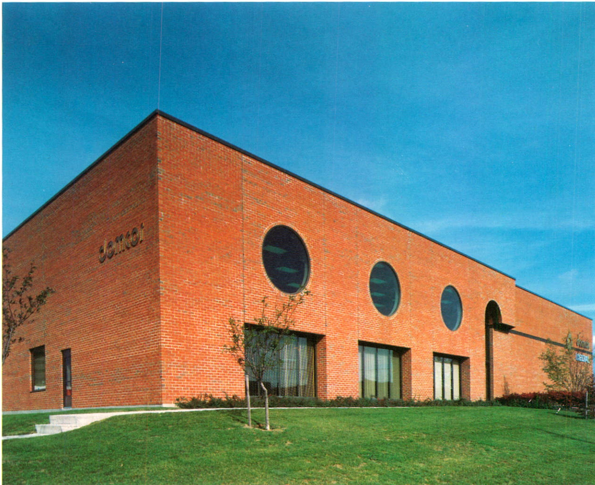
One of the 10 Domcor Distribution Centres
