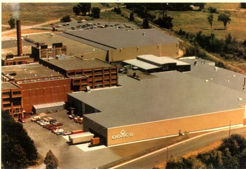
The Domco mill located in Farnham, Quebec.
