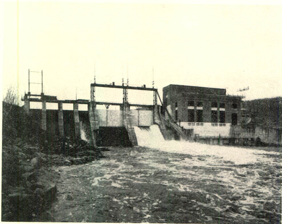
View from below the dam
